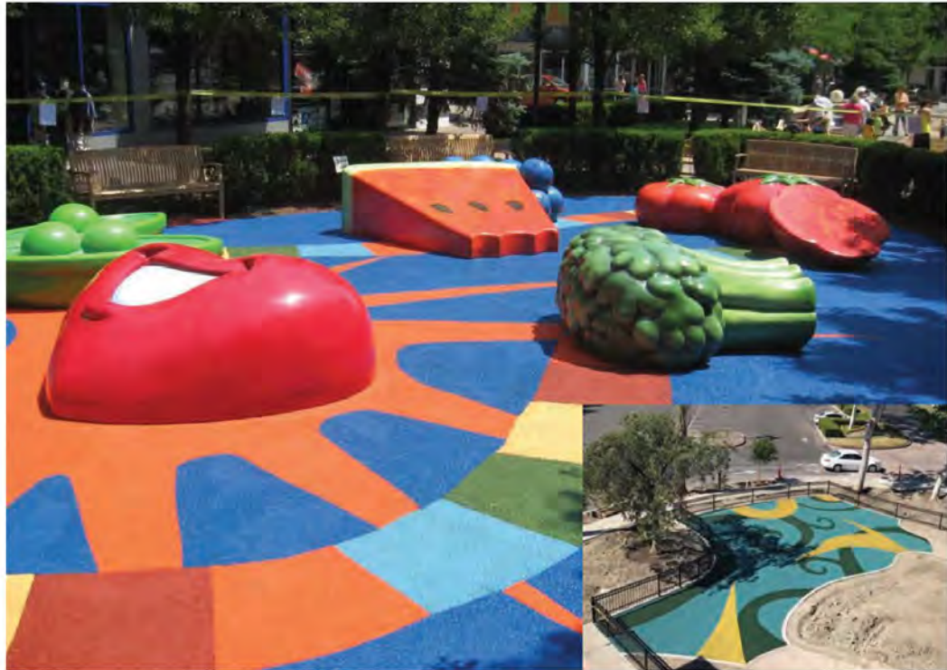
Poured in place rubber is durable, easy to clean, and ADA friendly. It also allows for unique and colorful designs which can help differentiate the children’s play space from the other, quieter dedicated spaces.
